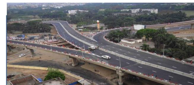
Mayor Mohammad Hanif Flyover (Completed October 2013)
