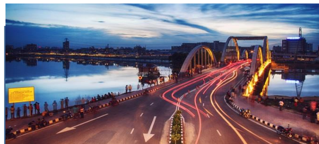
Hathirjheel – Begunbari Development (Completed January 2013)
